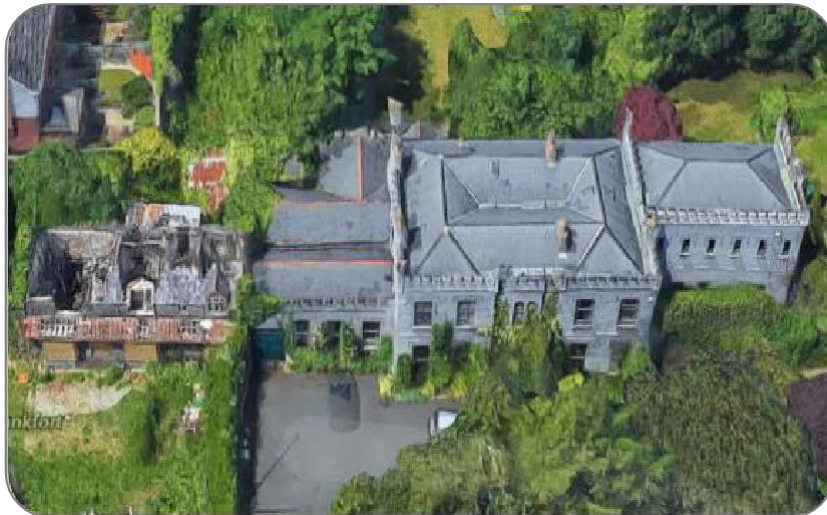
Figure 4-2 Aerial View of Existing Buildings 1-4 (image source: Google Map 2020)
